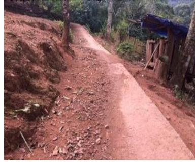
A section of Ngai Cho upgraded road with earth spillage on the road surface due to slope erosion in Phin Ho commune
